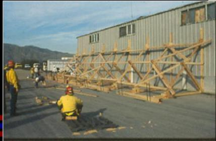
A photograph showing a large, complex wooden raker shore structure erected against a building under construction. Two workers in safety gear are visible near the base of the structure. The scene is outdoors with a clear sky and some distant hills.
